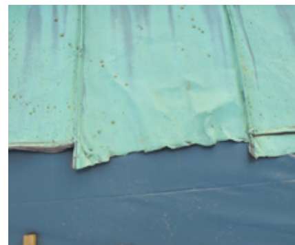
All Saints, Stretford, Manchester, stripped of its copper sheet roofing and (right) a close-up showing how they cut and removed the copper sheet (Photo: Angus Brown)
