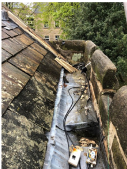
St Bartholomew's, Colne; (left) the uplifting of the lead flashing and external lighting cables which had been ripped up, and (right) a close-up of the damage caused to flashing and stonework (Photo: Angus Brown)
