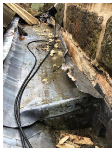
St Bartholomew's, Colne; (left) the uplifting of the lead flashing and external lighting cables which had been ripped up, and (right) a close-up of the damage caused to flashing and stonework (Photo: Angus Brown)
